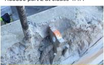
The erection design engineer may redesign the lift using an alternative to the damaged cast in lifter, such as this one, but it must be amended on the shop drawings and authorised by the erection design engineer.
