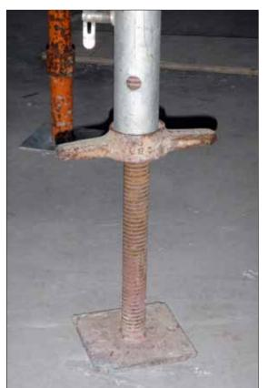
The minimum dimensions of a non-adjustable base-plate must be 150mm x 150mm, with a minimum thickness of 6mm. Attached to the centre of the upper surface of the base plate, there must be a shank or spigot not less than 50mm long and not less than 16mm in diameter (as per Australian Standards 1576.2 and 4576).
